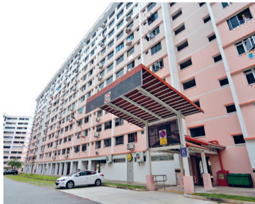
COMPLETED REPAIR AND REDECORATIONS AT BLKS 933 - 980
