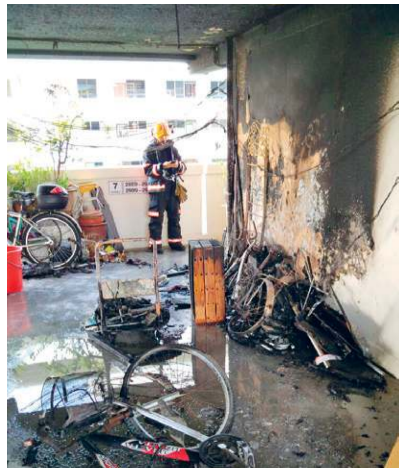
7 April 2016: fire involved items placed at the corridor in Eunos Crescent.
