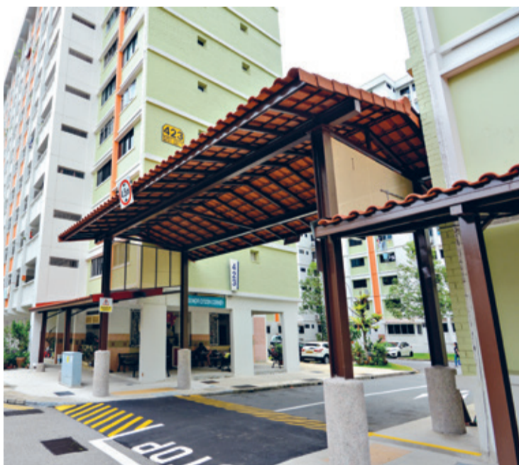
COMPLETED LINKWAY BETWEEN BLK 422 AND 423
