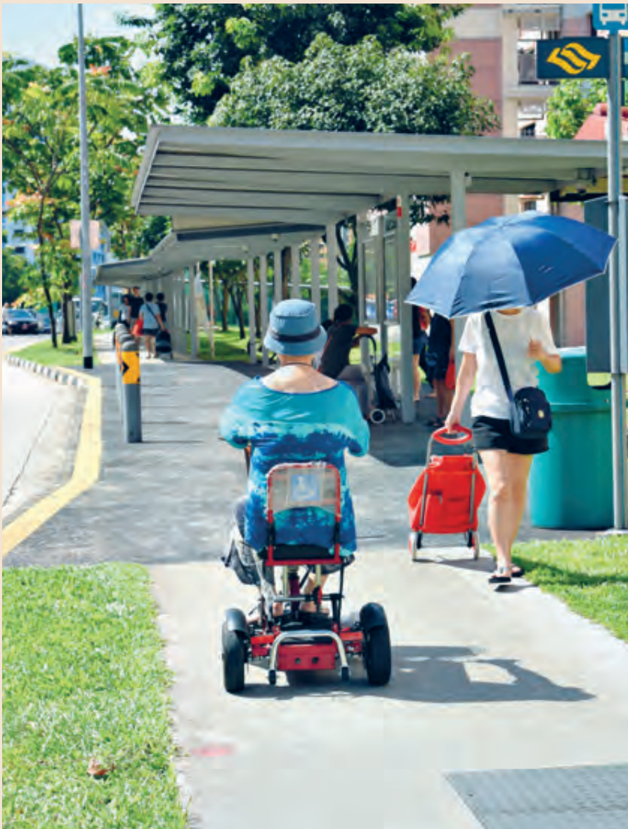
Widened Footpath at Pioneer Road North Community Garden between Block 942 and Block 945
