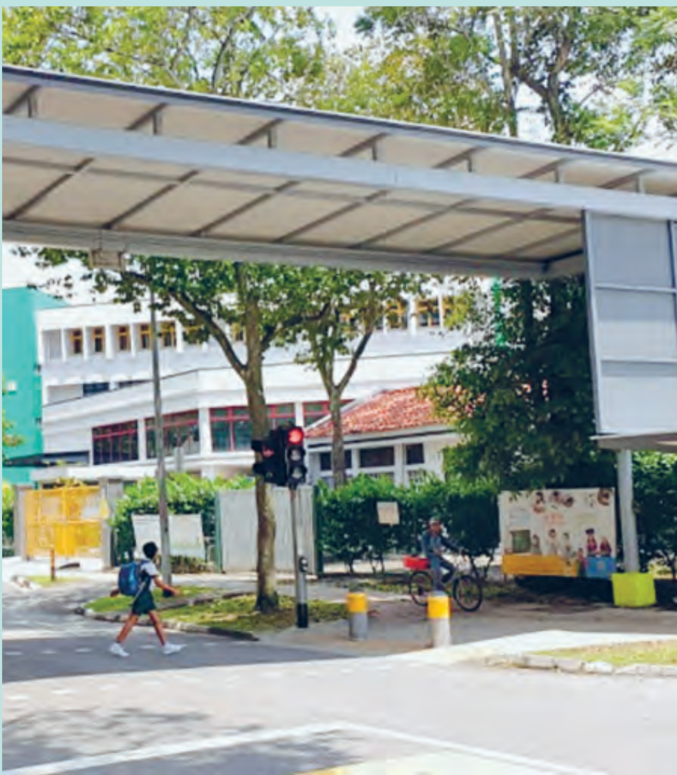
Block 920 to traffic light junction outside Juying Primary School
