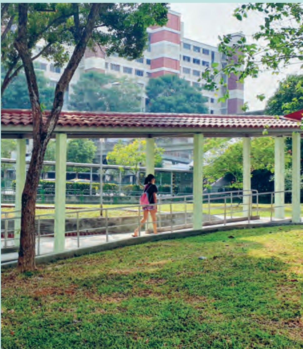
Covered Walkway at Block 840 to Block 845
