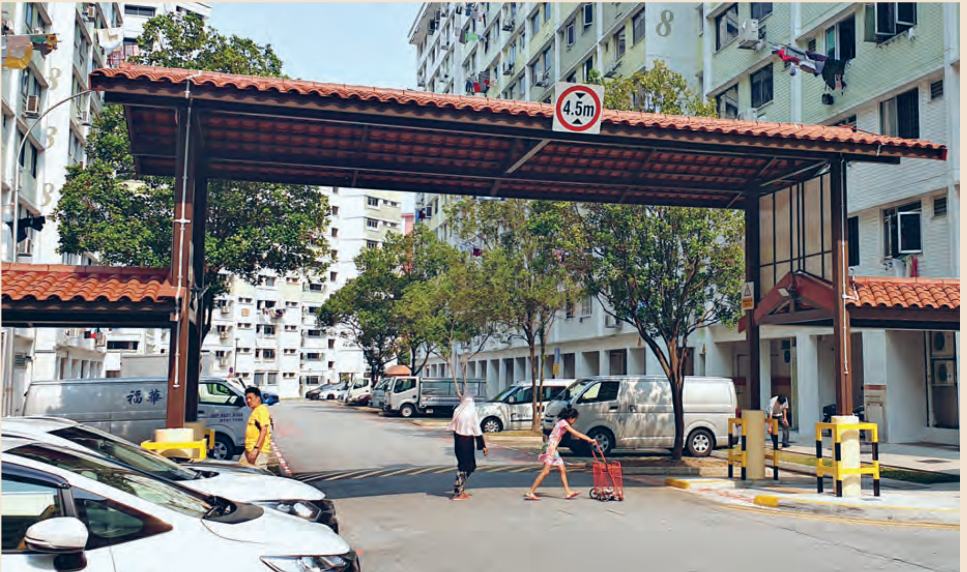
Covered Walkway at Block 835 to Block 838
