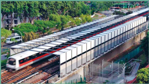
SOUND BARRIERS (COVERING UP TO 2,900 METRES) Installed along MRT viaducts, these barriers aim to reduce noise levels.
