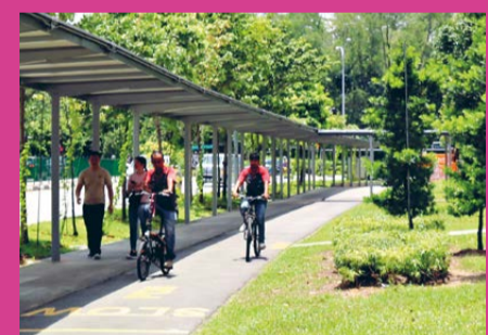
WIDENED FOOTPATH AND CYCLING PATH A new 8.6-kilometre route for cyclists to explore.
