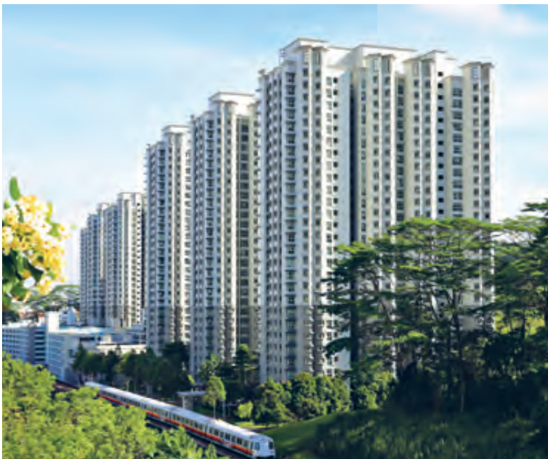
Repairs and Redecoration Programme
