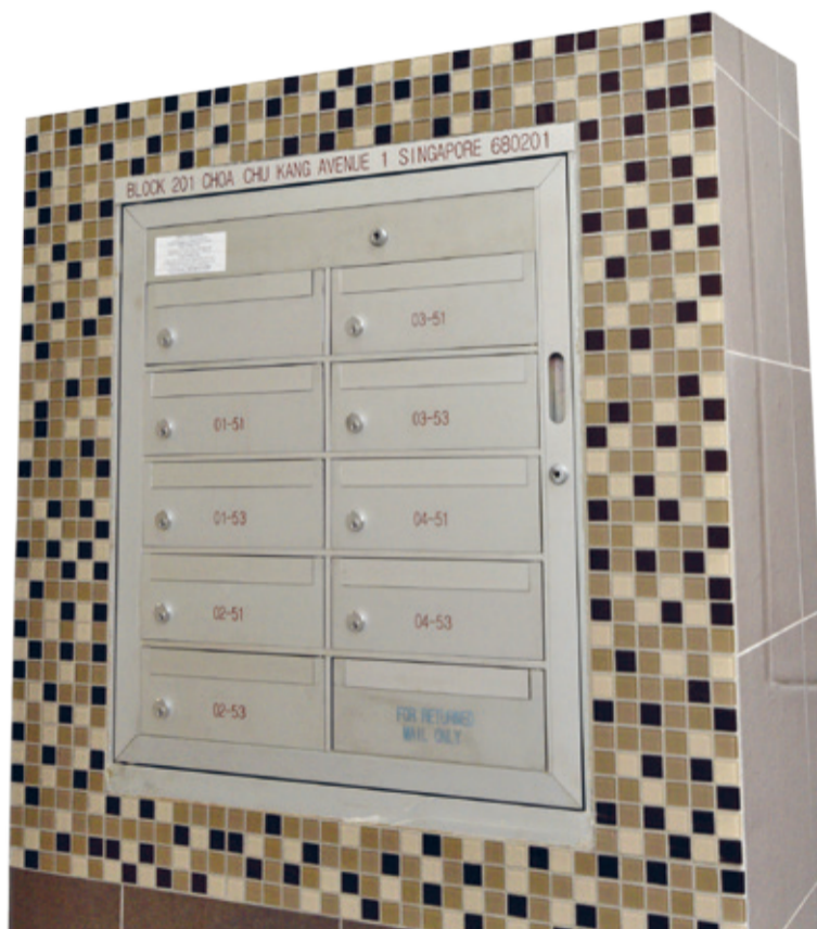
COMPLETED UPGRADED LETTERBOXES AT BLKS 201 - 221 AND BLKS 223 - 239
