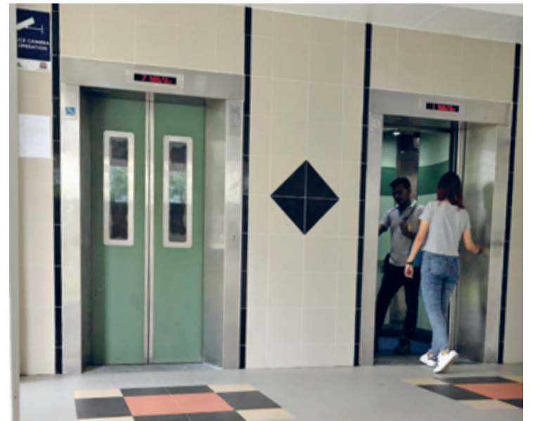
COMPLETED LIFT UPGRADING AND LIFT REPLACEMENT
