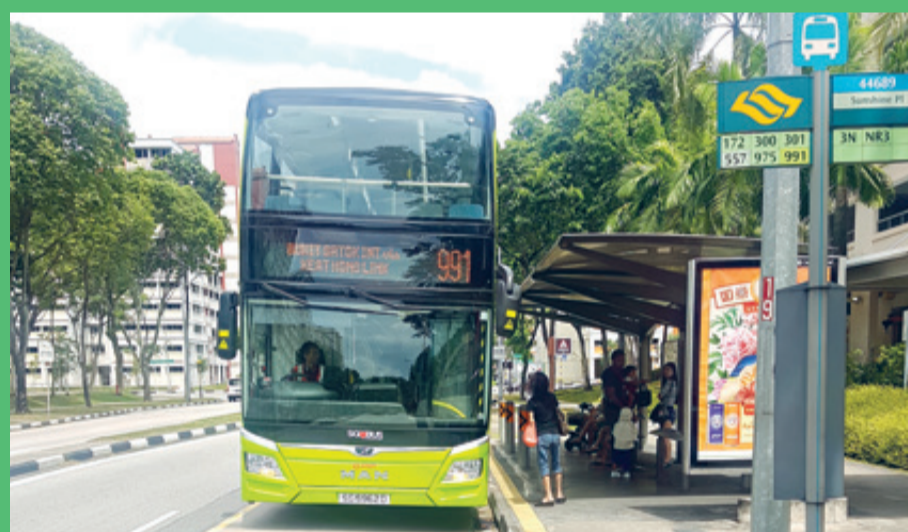
MRT Sound Barrier Construction works for a noise barrier installation have commenced to reduce noise generated from trains running along the MRT track.
